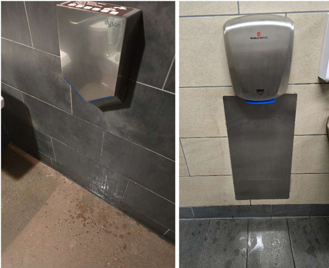
Figure 4. Water dispersion patterns in dispersal-type hand dryers. Dyson Airblade (left) and World Dryer VerdeDri (right) installations showing characteristic plume patterns on walls and floors beneath devices. Water displaced from hands during operation settles on surrounding surfaces rather than evaporating. Manufacturer documentation contains zero statements addressing water destination after air jets strike it.
